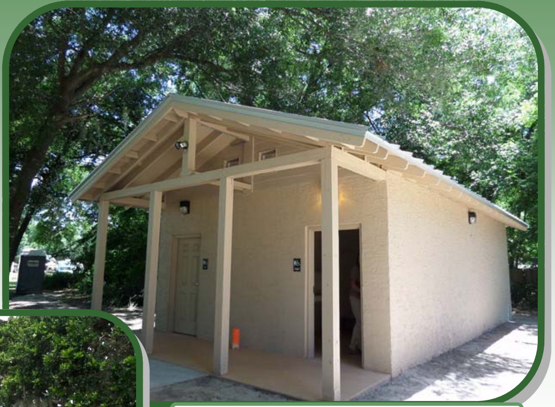
Cadwell Park Restroom Facility
